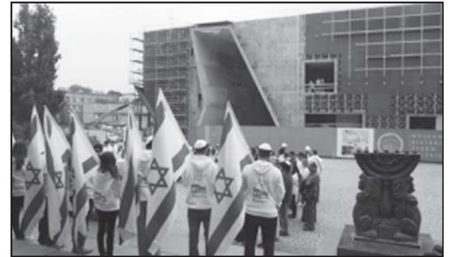
Young Israelis stand in front of the building under construction for the Museum of the History of Polish Jews in Warsaw, Poland.
